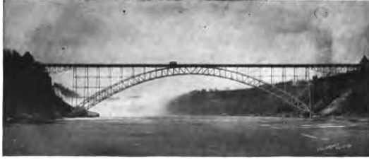
Bridge over the Niagara River, connecting Niagara Falls, New York, with Clifton, Canada. New York Approach Span, 190 feet long. Canadian Approach Span, 210 feet long. Main Span, 840 feet long. The Roadway is 185 feet above water line. Total structure weighs 2,239 tons. Built for the Niagara Falls and Clifton Bridge Company by the
