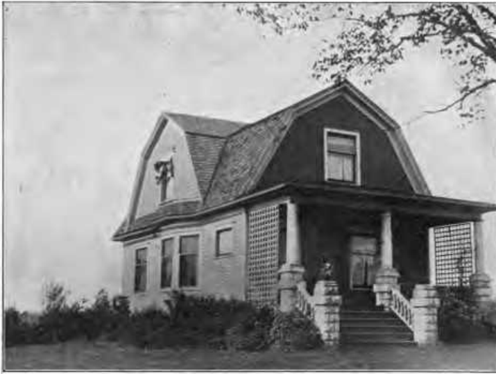
Masses of hardy shrubs about the foundation of the house tend to harmonize it with its site.
