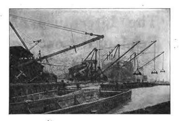
Handling Sand, Gravel and Crushed Stone in the construction of the Pittsburgh Filtration Plant, Aspinwall, Pa.
